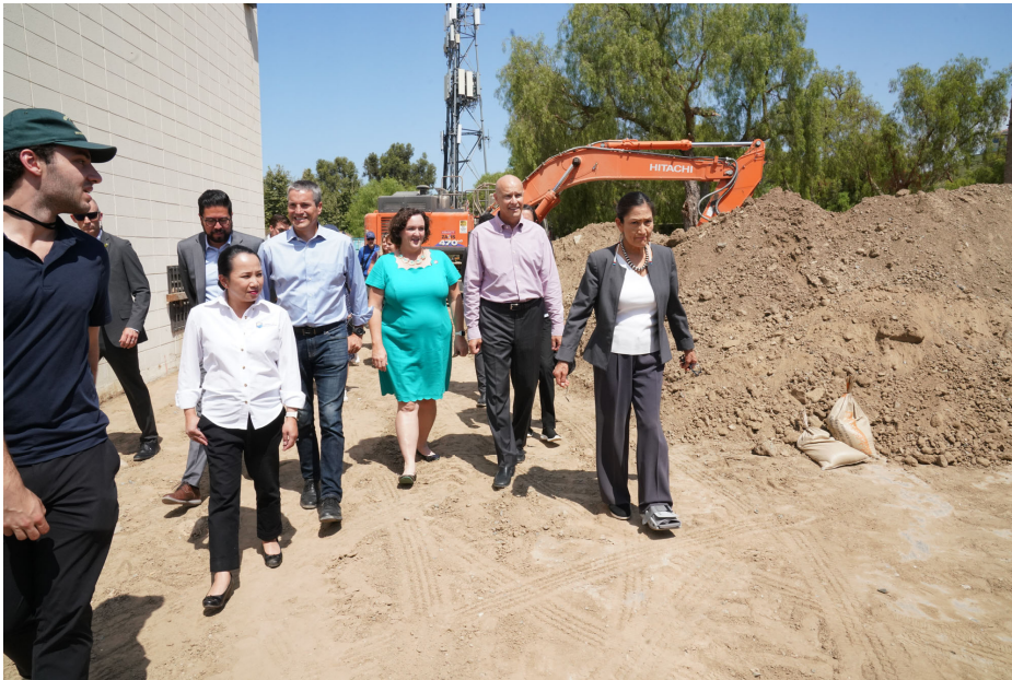
Secretary Deb Haaland and Commissioner Camille Touton tour Irvine Ranch Water District's Syphon Reservoir Improvement Project in Irvine, CA, August 2022. Reclamation IJA funding of $12.2 million for this project, FY 2022.
